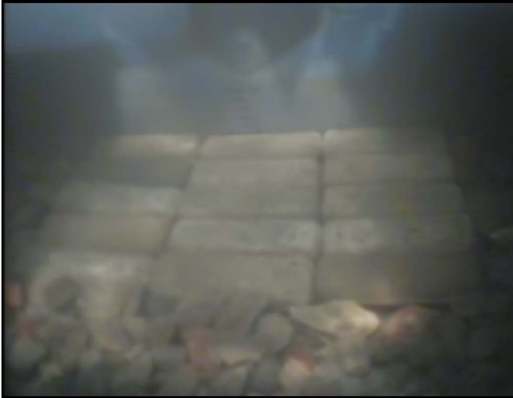
Figure 32 - 14,000 lb grout-filled bags in place after testing at 370 ft. elevation
