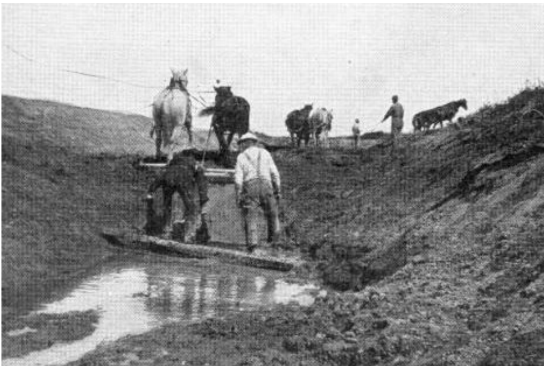
Figure 32: Construction of a Drainage Ditch by Horse and Plow in Minnesota, 1908
