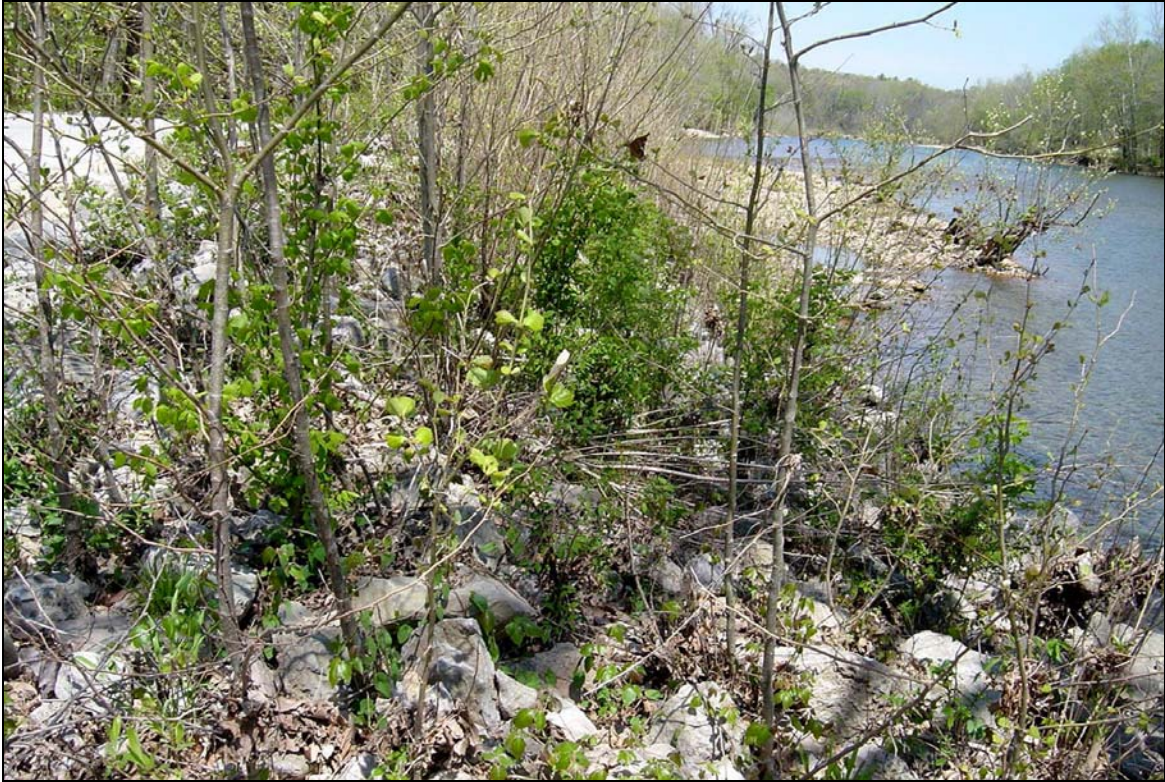
Figure 77: Willow Plantings and Rock Revetment for Erosion Control
