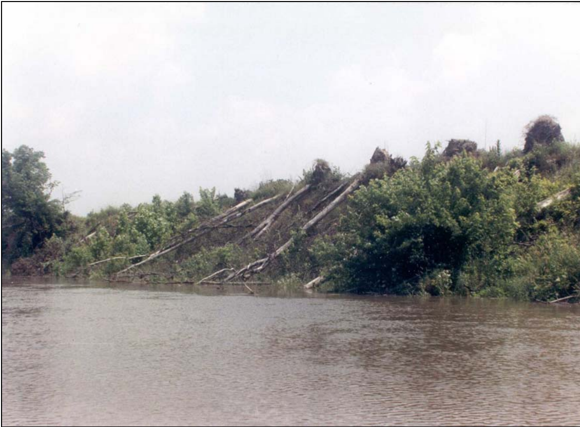
Figure 82: Anchored Cut Trees for Bank Erosion Control on the Salt River in Central Missouri (Rapp 2005)
