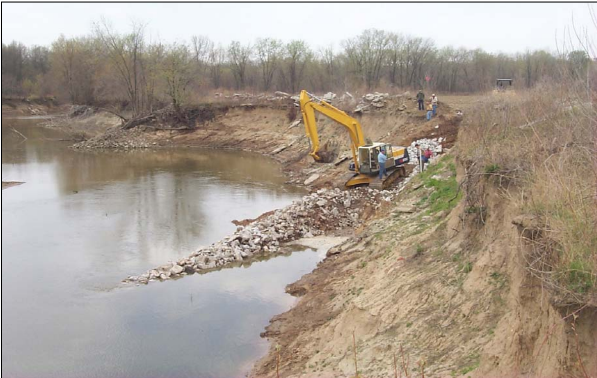
Figure 81: Rock Vane Construction for Bank Stabilization on the Kaskaskia River
