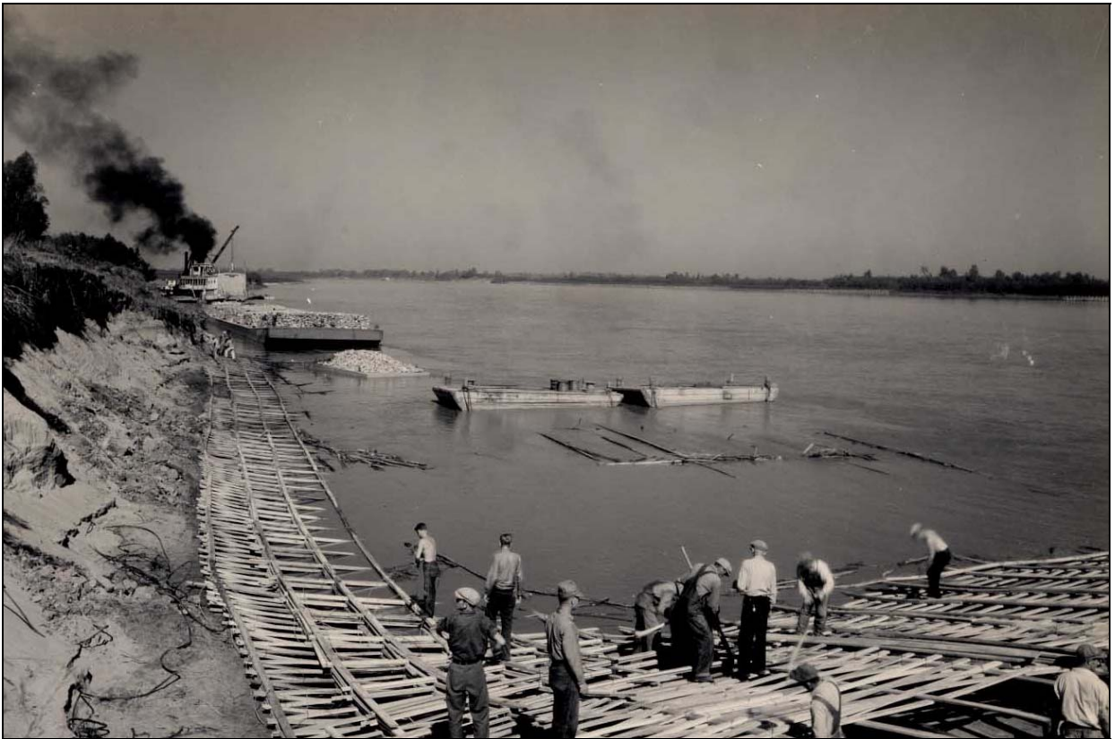
Figure 79: Wooden Mattress Placed along an Eroding Bank of the Mississippi River (Circa 1938)
