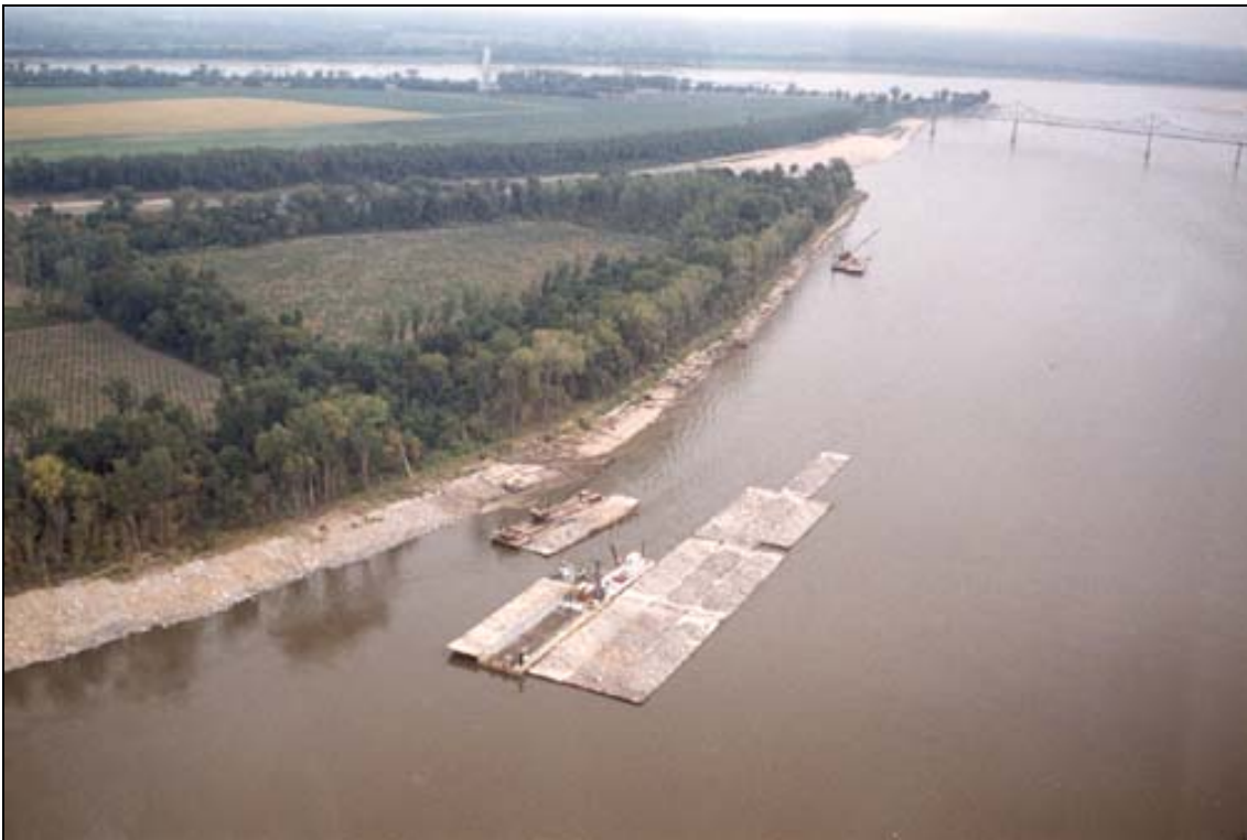
Figure 75: Revetment Being Placed along the Bankline of the Mississippi River
