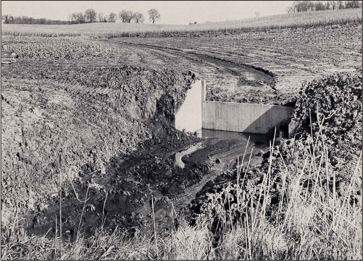
Figure 83: Concrete Grade Control Measure near Iowa City, Iowa
