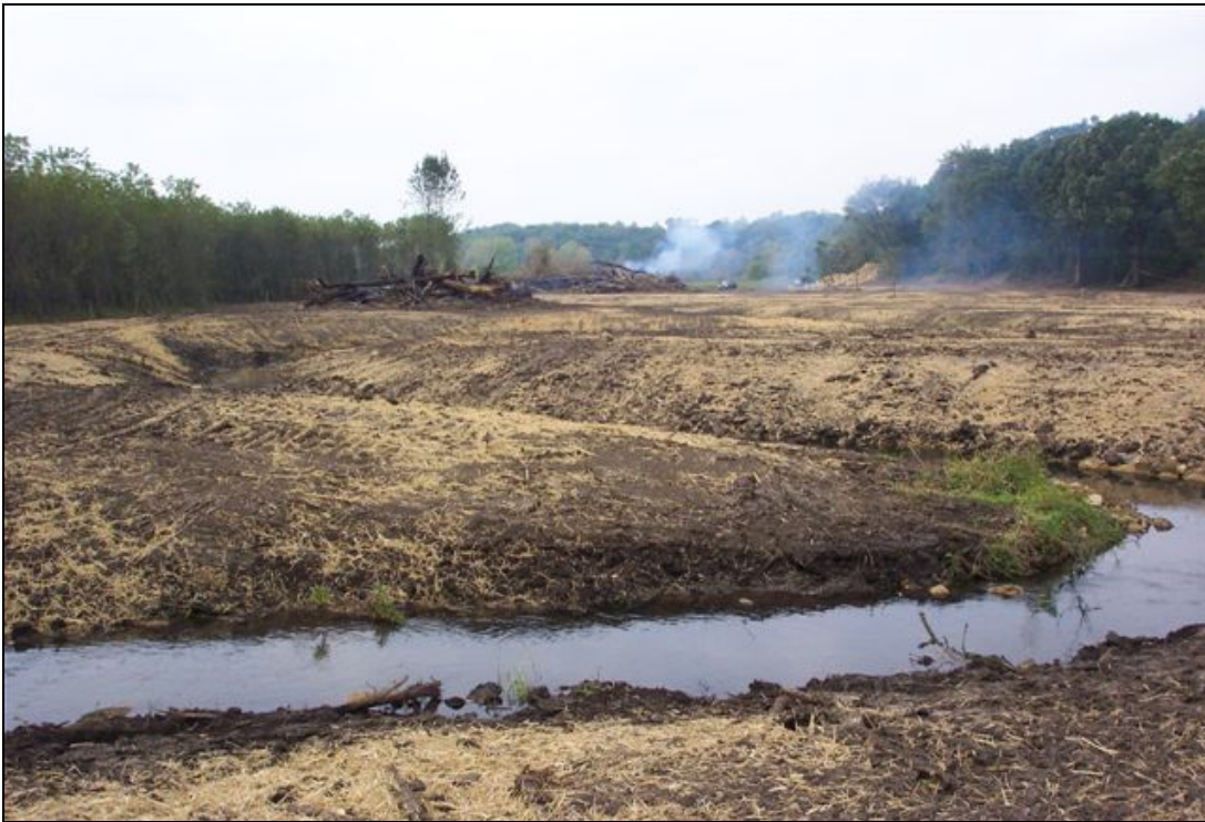
Figure 88: Earth Moving and Vegetation Removal of the Floodplain along the Gordon River (West 2005)
