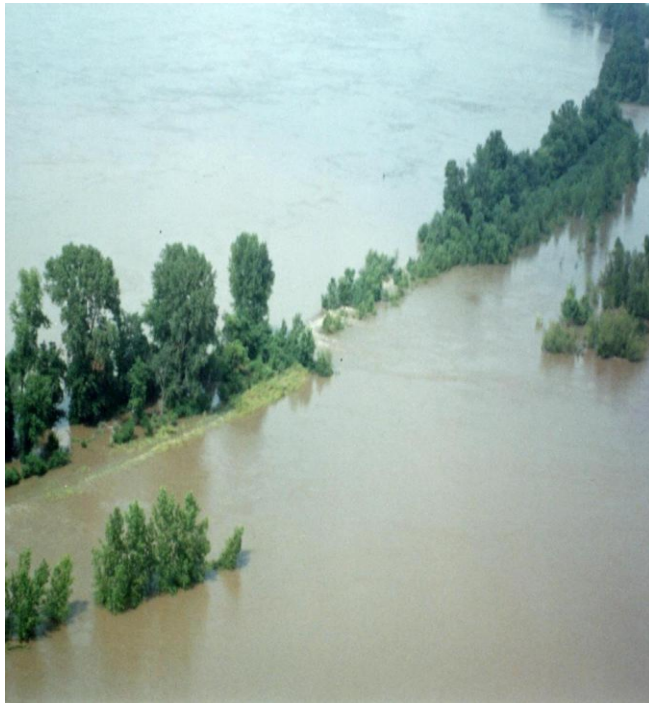
Figure 14: Hillhouse Break 4 During 1993 Flood
