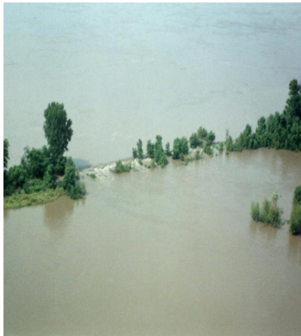
Figure 12: Hillhouse Break 2 During 1993 Flood
