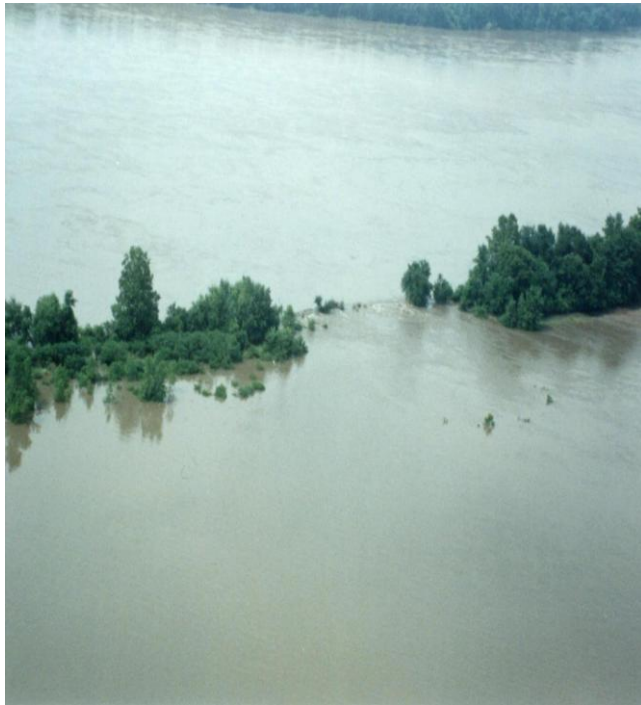
Figure 13: Hillhouse Break 3 During 1993 Flood
