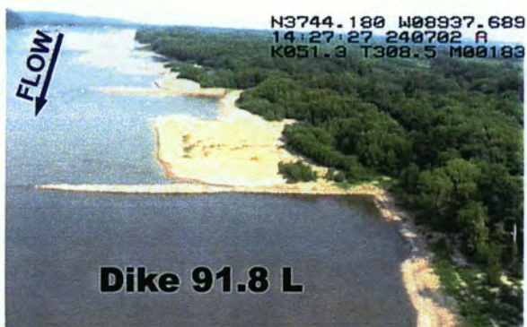
Dike 91.8 L Dike height is +19 to +12 Ft. LWRP Approximate length is 500 Ft.
