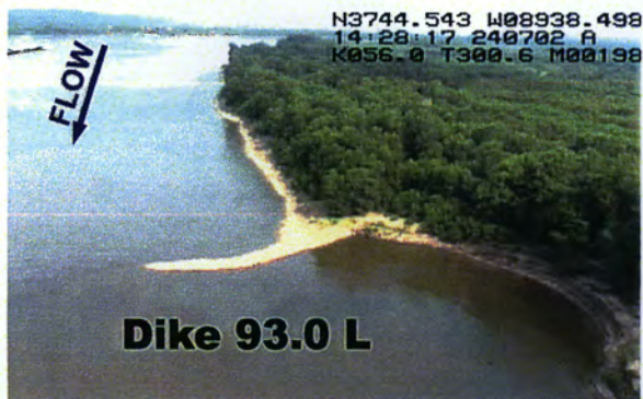
Dike 93.0 L Dike height is +16 Ft. LWRP Approximate length is 250 Ft.
