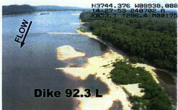
Dike 92.3 L Dike height is +16 Ft. LWRP Approximate length is 350 Ft.
