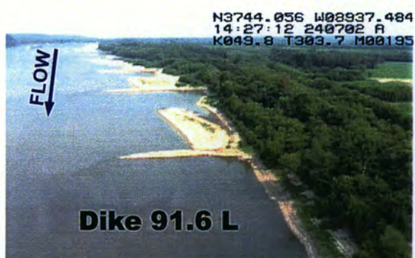
Dike 91.6 L Dike height is +12 to +10 Ft. LWRP Approximate length is 300 Ft.
