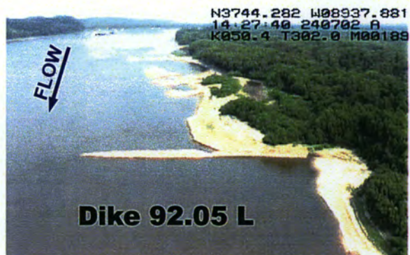
Dike 92.05 L Dike height is +16 Ft. LWRP Approximate length is 490 Ft.
