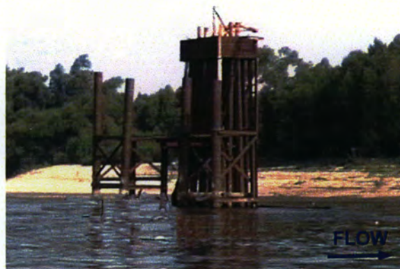
Abandoned Loading Facility Located Along the LDB at Mile 85.6
