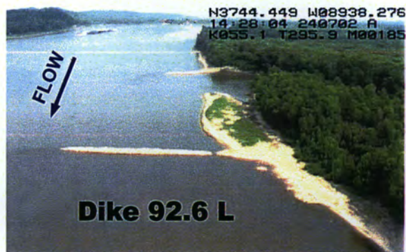
Dike 92.6 L Dike height is +16 Ft. LWRP Approximate length is 430 Ft.
