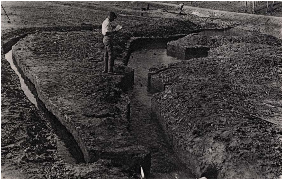
Figure 4. First Hydraulic Model at WES, Illinois River Model (from "History of WES")
