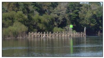
Wood Pile Structures - Prior to the 1960's almost all of the structures placed in the Middle Mississippi River were of the woody pile type. Logs were driven into the river bed to create roughness and formed into a river training structure. Due to the higher maintenance of these woody structures, river training structures began to be constructed from stone during the 1960s. There is currently a push to start bringing back the
