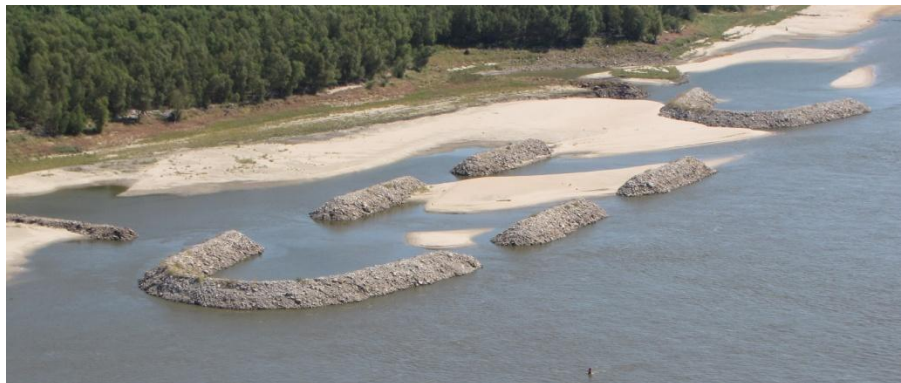
Exhibit 12. Observed flow and sediment patterns occurring at the Runway Chevron during summer 2012 sample. Photo taken on 24 September 2012. St. Louis gage -2.5 feet.
