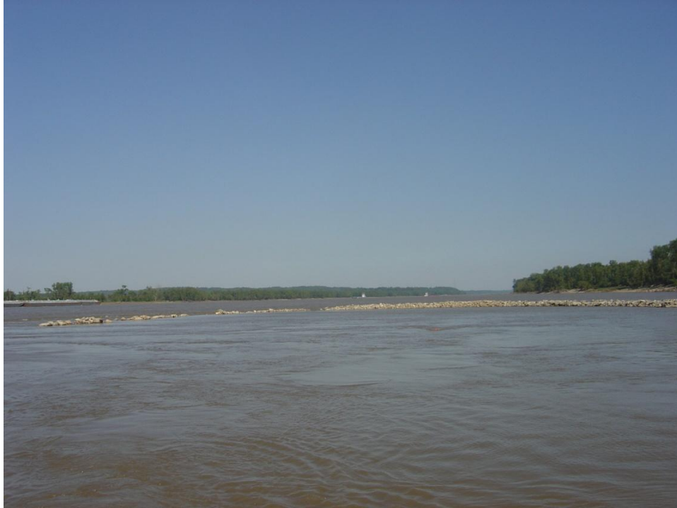
Photo 2. Navigation side left of chevron in the Runway Chevron Field (RM 36) partially submerged. Thebes gage at 17.35 feet. April 30, 2012.
