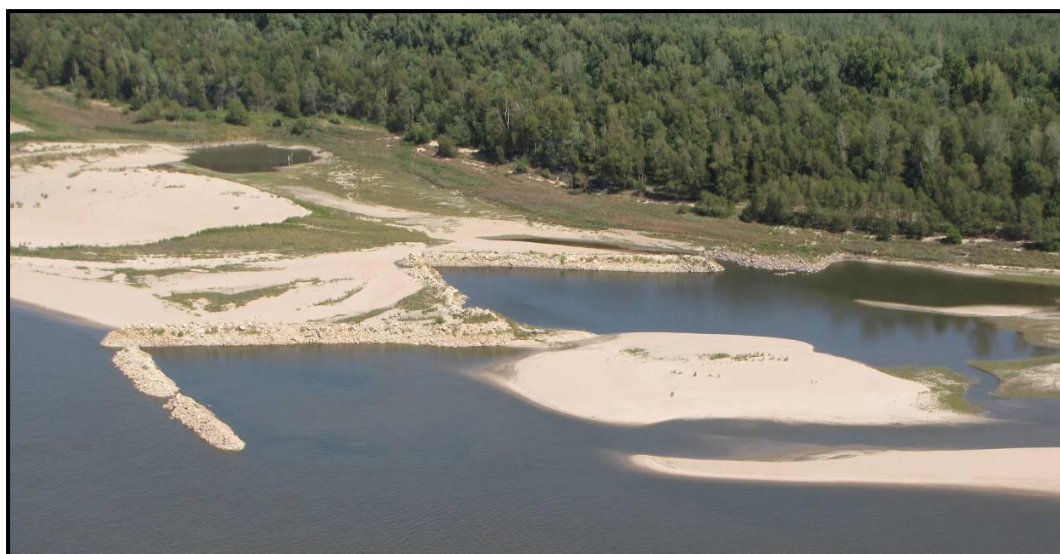
Photo 3. Aerial view of the W-Dike taken on 24 September 2012 during low water conditions. Notice the large area of accretion upstream and downstream of the structure.
