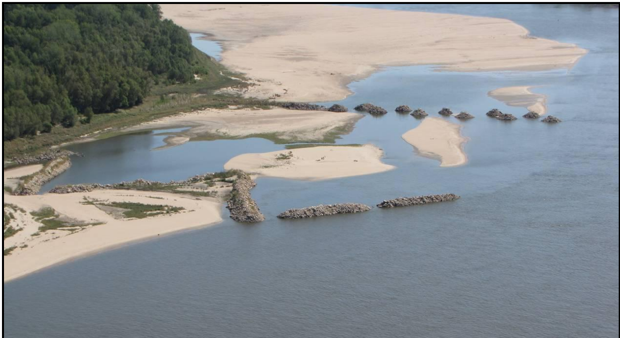
Photo 4. Aerial view of the W-Dike and MRS structures taken on 24 September 2012 during low water conditions. Notice the missing sections of rock within the W-Dike. Although not designed into the structure, these areas allow additional scour to occur.
