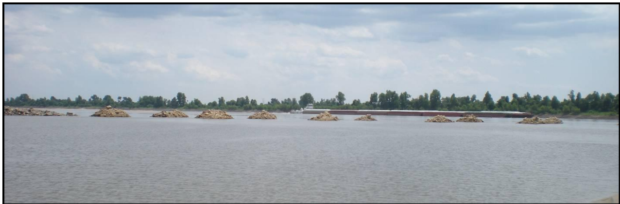
Photo 1. View of Multiple Round Point Structures (MRS) looking downstream.
