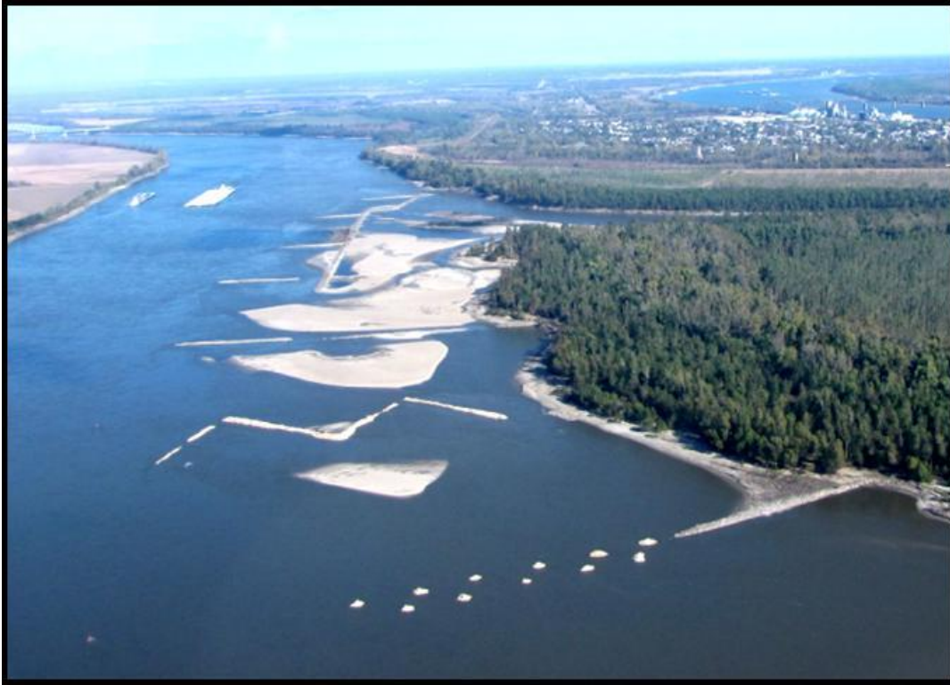
Photo 2. Aerial view of the experimental site, taken on 5 November 2012, showing the MRS, W-dike, and notched dike.
