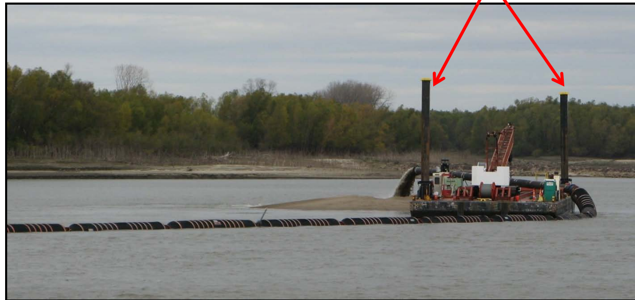
Flexible Floating Pipe attached to rigid pipe fixed to the Temporary Spill Barge
