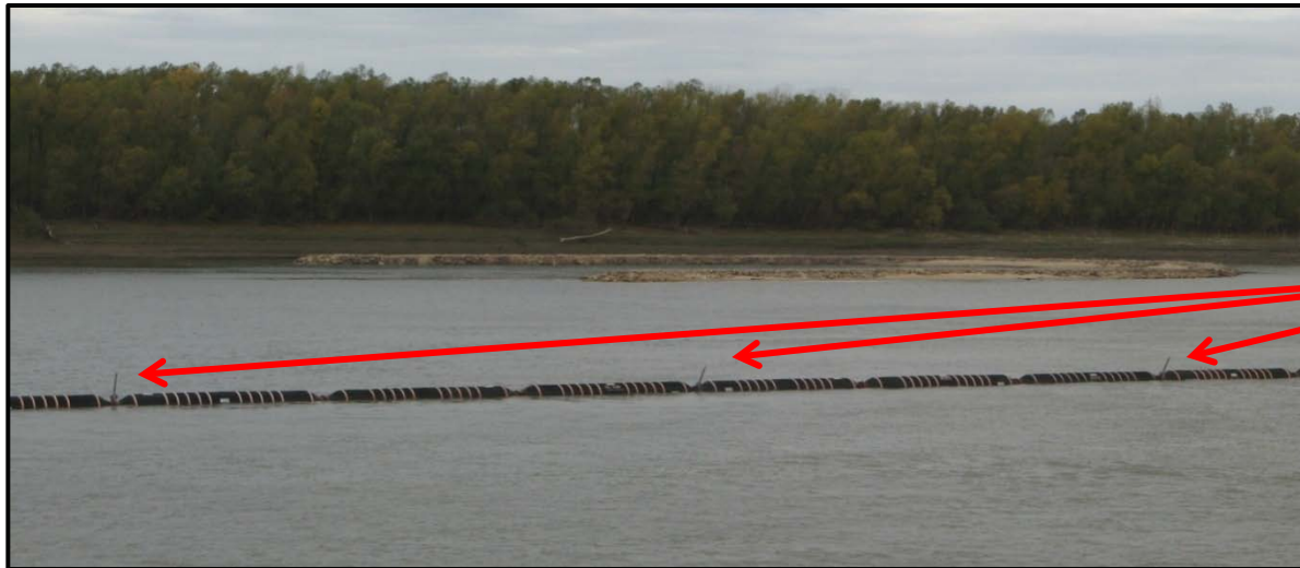
Flexible Floating Pipe with intermittent attached lights
