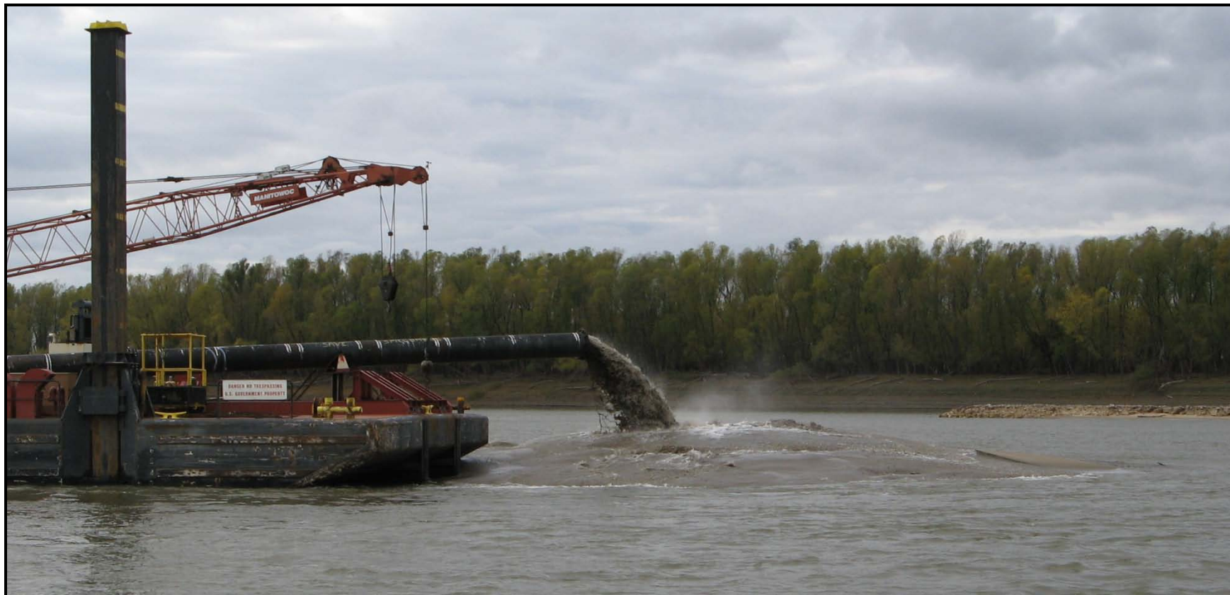
Formation of Island/Bar using Dredge Disposal
