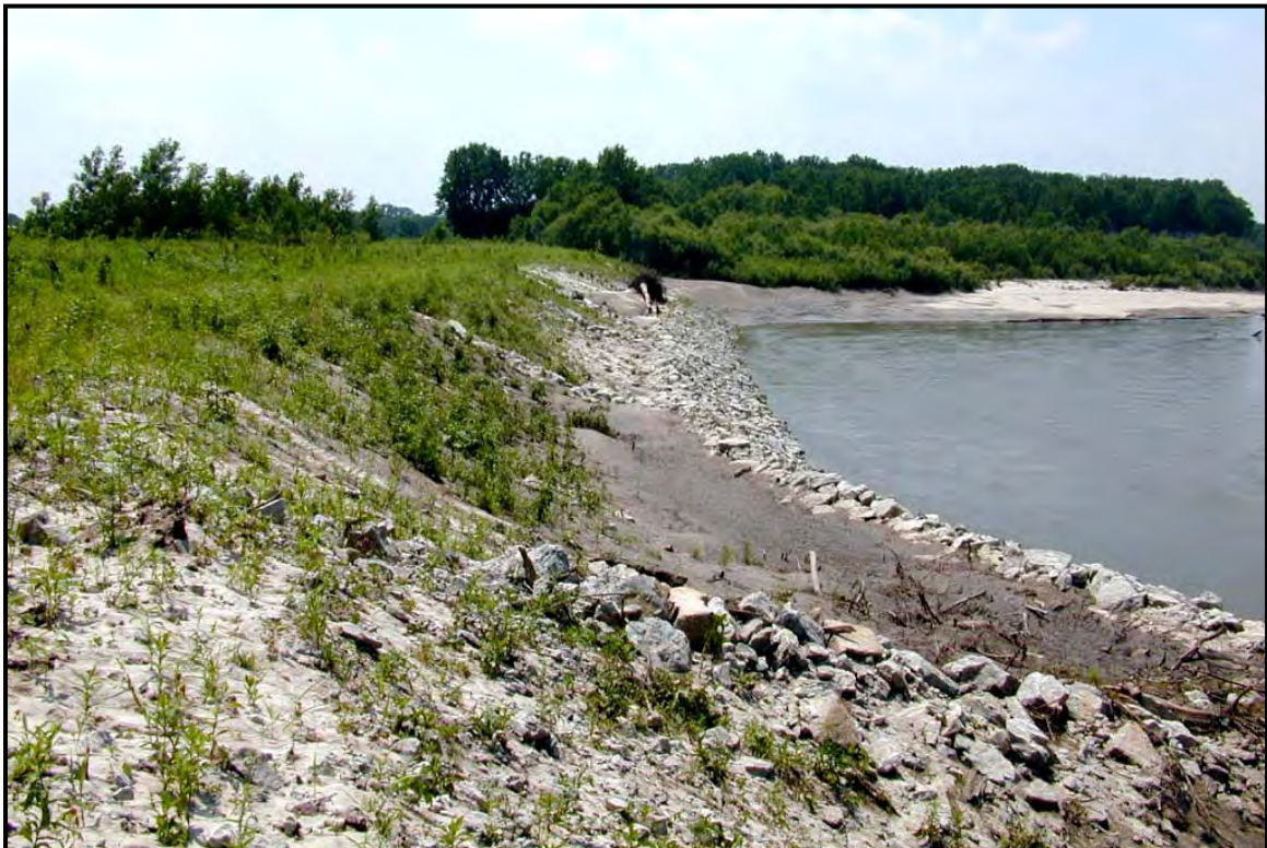
Picture 7. LPSTP Three Months Post Construction (notice sedimentation & vegetation)
