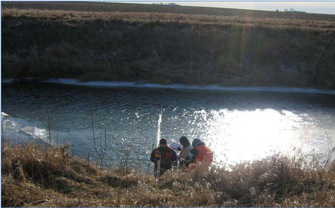
Picture 2. Typical Upper Reach Channel Section
