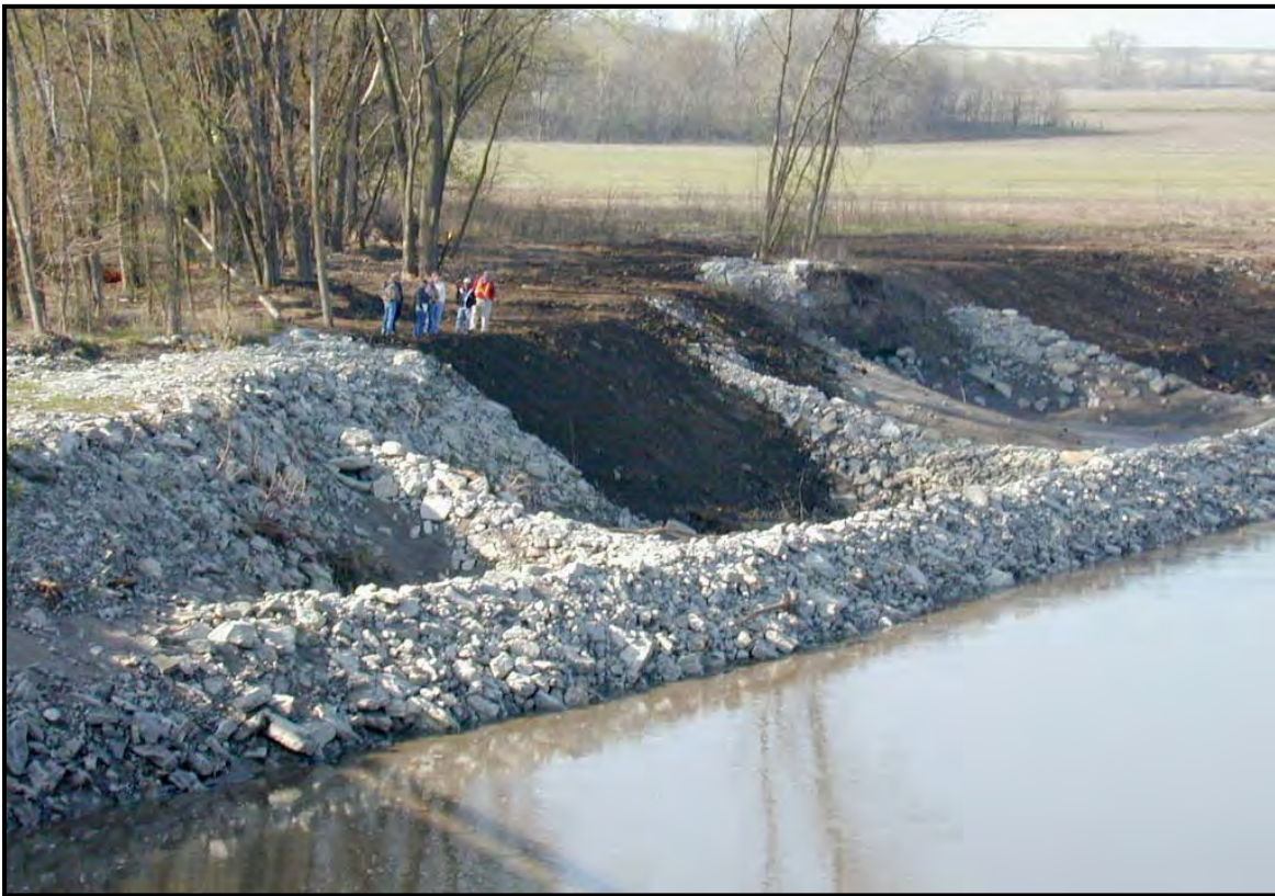
Picture 6. LPSTP Immediately Post Construction
