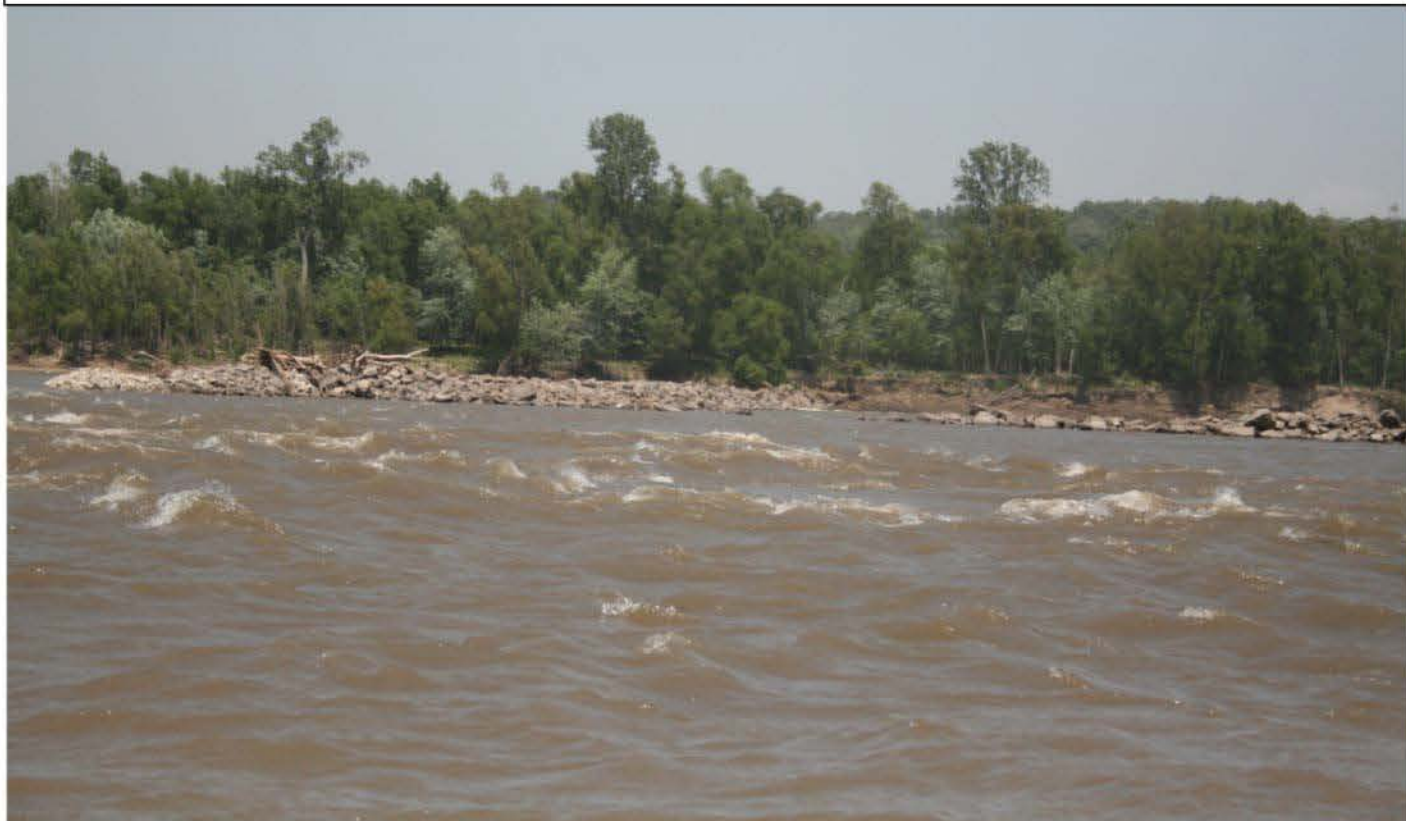
Looking downstream at Dike 39.60L – This dike is located at the entrance of Santa Fe Chute and keeps most flows from entering the side channel unless there is higher water. The dike has a low spot at which water at low stages can get through. The photo above was taken on April 18 while the photo below was taken May 24, both showing the dike at its low spot. The side channel is mostly very shallow as seen on the 2011 aerial photograph (photo to the right).
