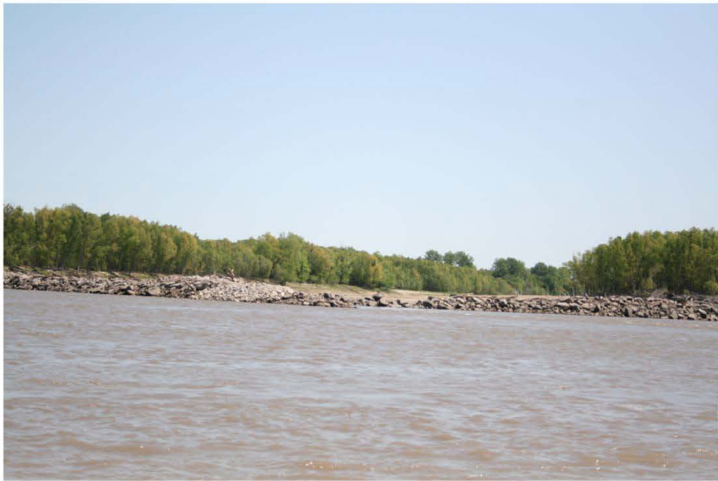
Looking downstream at Dike 39.60L – This dike is located at the entrance of Santa Fe Chute and keeps most flows from entering the side channel unless there is higher water. The dike has a low spot at which water at low stages can get through. The photo above was taken on April 18 while the photo below was taken May 24, both showing the dike at its low spot. The side channel is mostly very shallow as seen on the 2011 aerial photograph (photo to the right).
