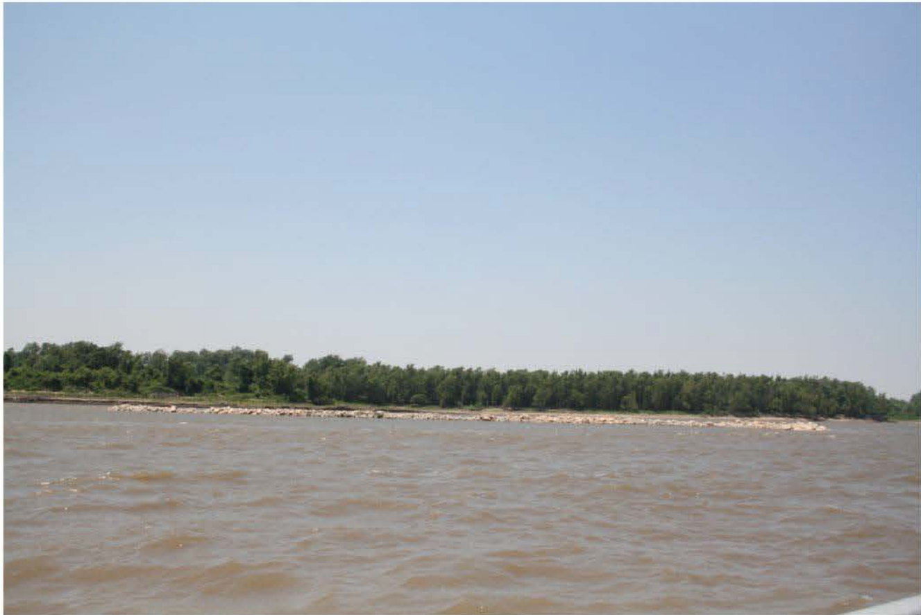
Looking upstream at Chevron 32.60 R (left photo) & Chevron 32.80R (right photo) — There is a difference in height between the right and left leg of the chevron, the left leg is lower on both. Chevron 32.40R was in good conditions.
