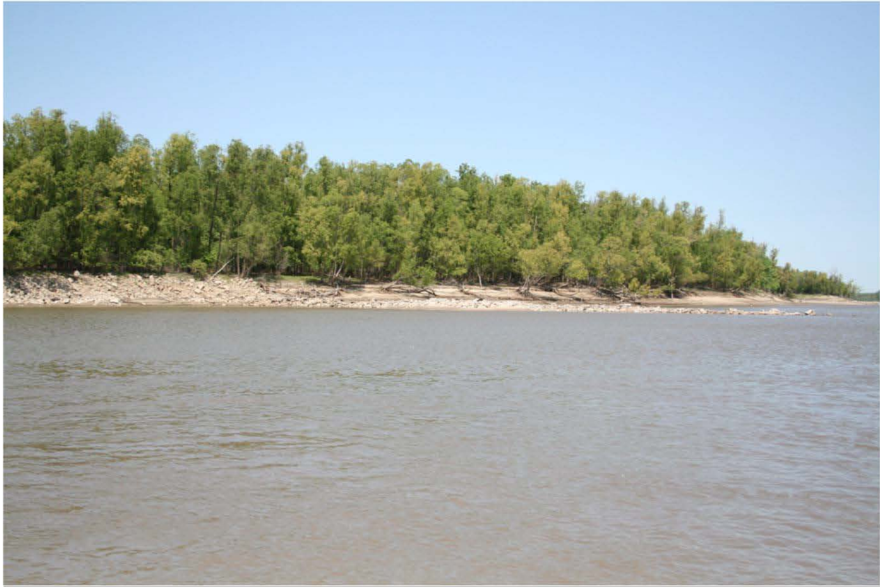
Looking downstream at Dike 32. 20 L - Most dikes and banklines appeared to be in fairly good conditions.
