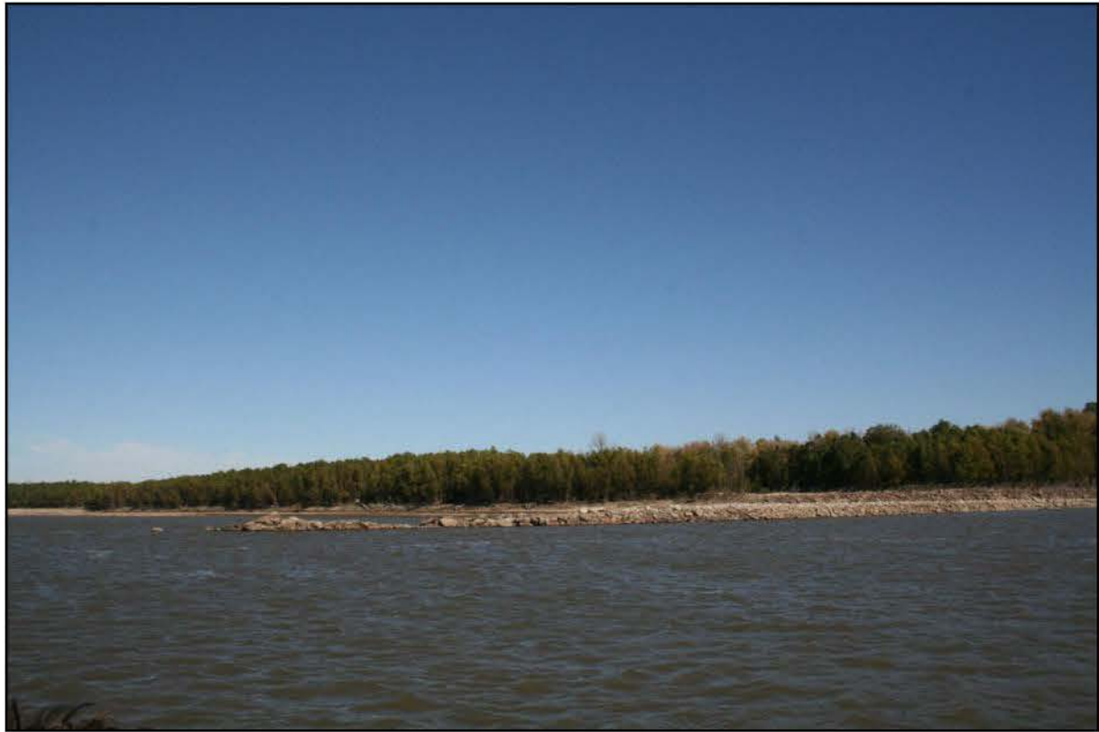
Photograph 1: Looking upstream at Dike 67.30 along the LDB
