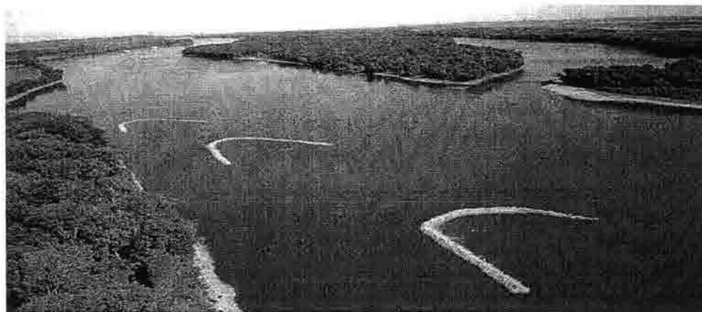
Figure C. Chevron dike field at Mississippi River mile 266. The deep slack water habitat formed behind these structures has been shown to be used extensively by fish in the winter.
