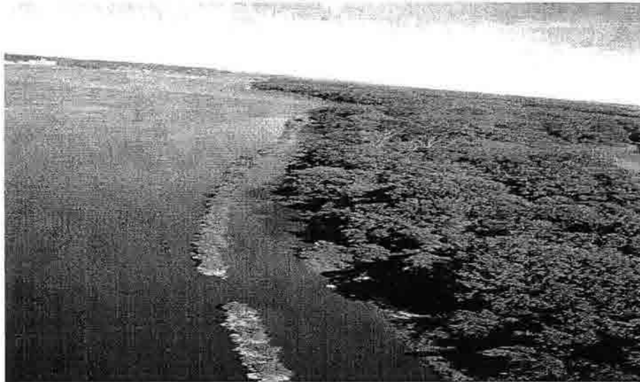
Figure E. Off-bankline revetment at Crider Island, Mississippi River mile 280. Note the notch in the structure to allow water exchange and angler and fish access.
