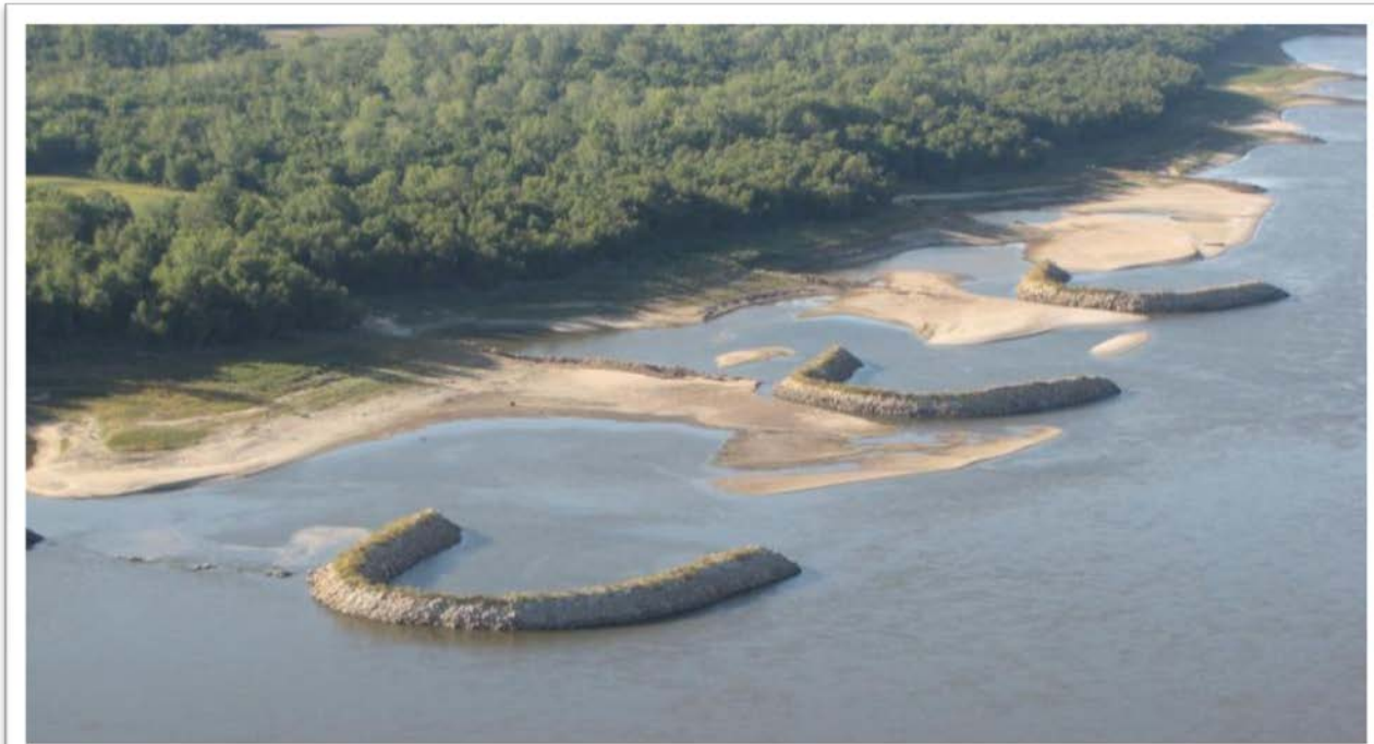
Cliff Cave – Kimmswick chevrons (RM 162L (top photo) and RM 160L (bottom photo)) during low-water fly-over September 2012 (river level -2.5 on St. Louis gage).
