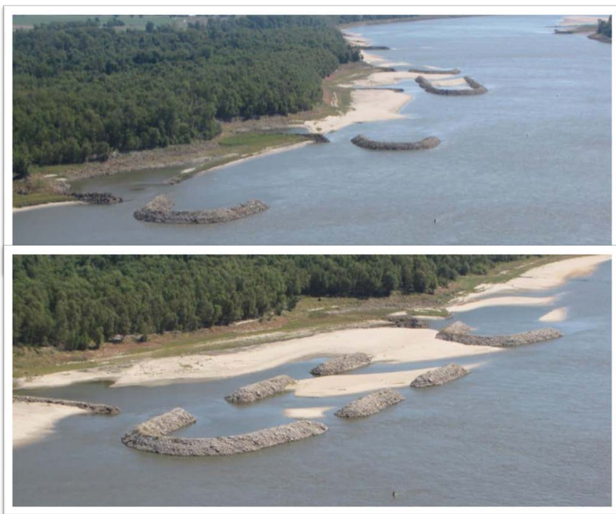
Dogtooth Bend chevrons (RM 36L) during low-water fly-over September 2012 (river level -2.5 on St. Louis gage).
