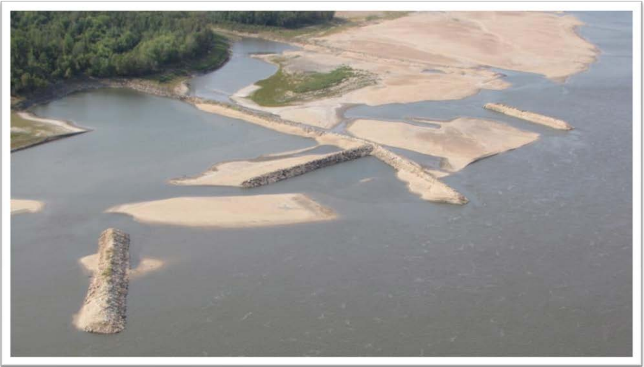
Vane dikes (RM 96R) during low-water fly-over September 2012 (river level -2.5 on St. Louis gage).
