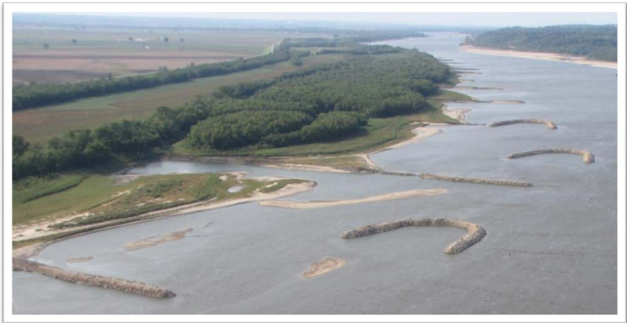
Waters Landing chevrons (RM 104R) during low-water fly-over September 2012 (river level -2.5 on St. Louis gage).
