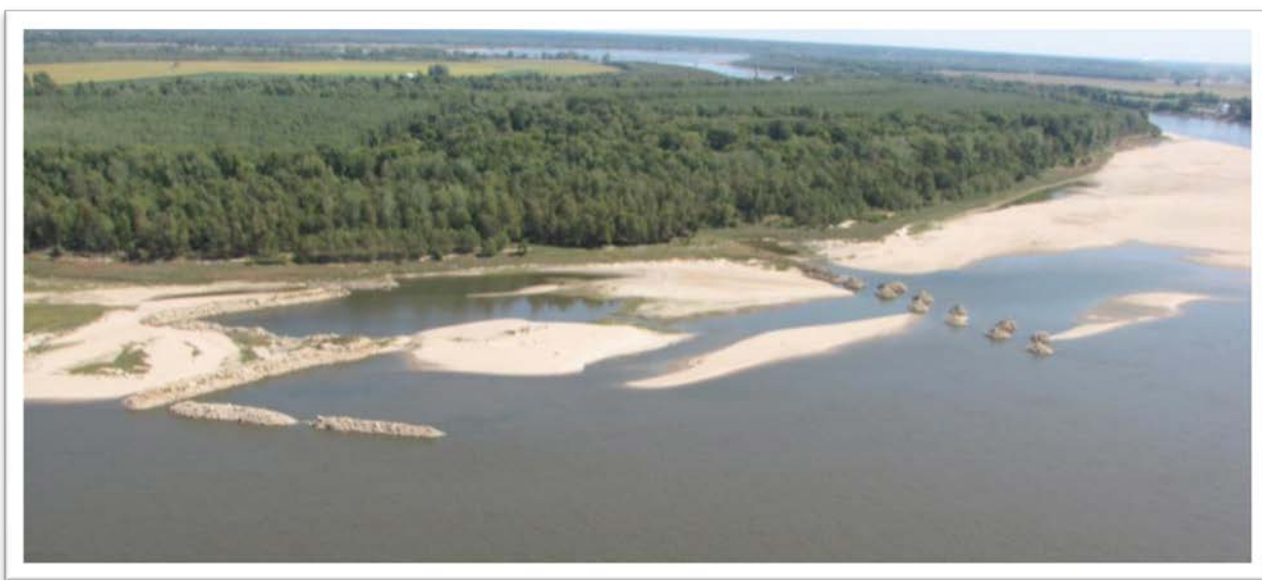
W-dike and multiple roundpoint structure (RM 4L) during low-water fly-over September 2012 (river level - 2.5 on St. Louis gage).
